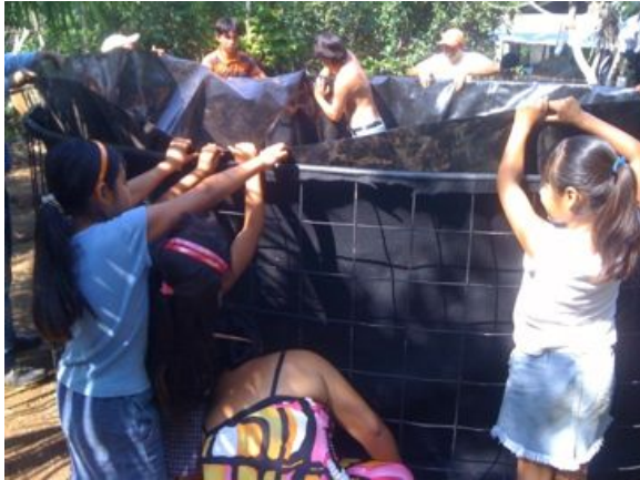
Assembling geomembrane tank for fish
